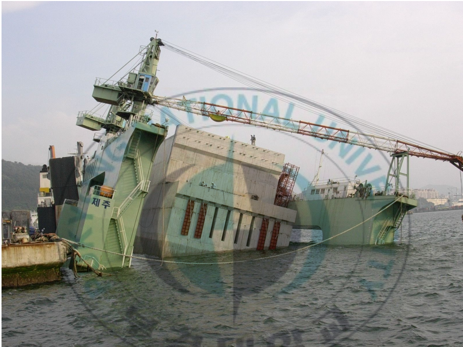
Fig. 1.1 Damage of produced caisson.
