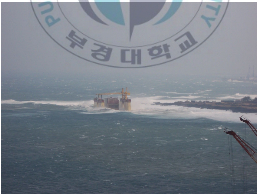
Fig. 1.3 Damage of Derangement Wave FD.
