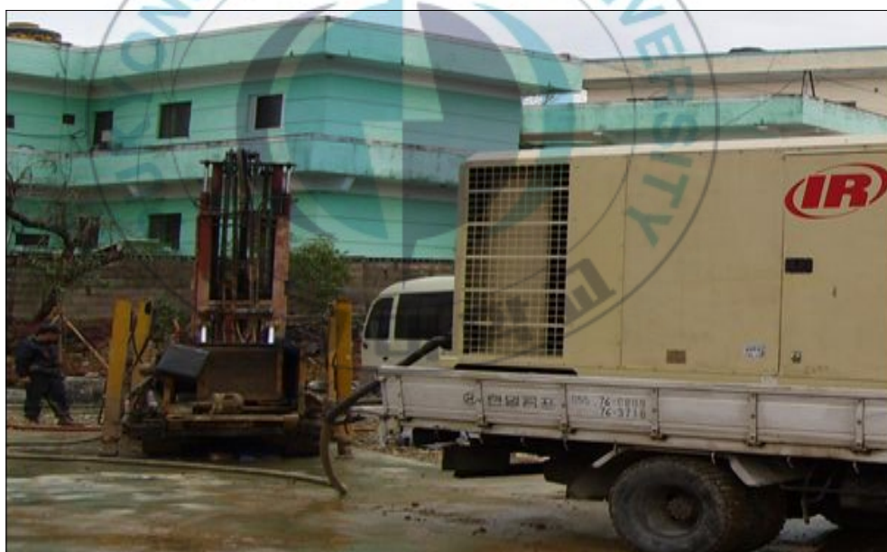
Fig. 16. Injection of high pressure air in the site.
