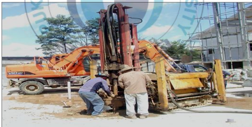
Fig. 3. Photography for the pilot scale test site taking soil cores and installing wells.
