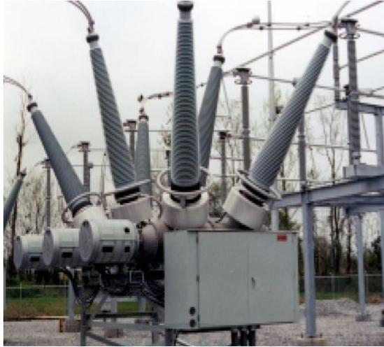
Fig. 2.2 Air pressure type circuit breaker.
