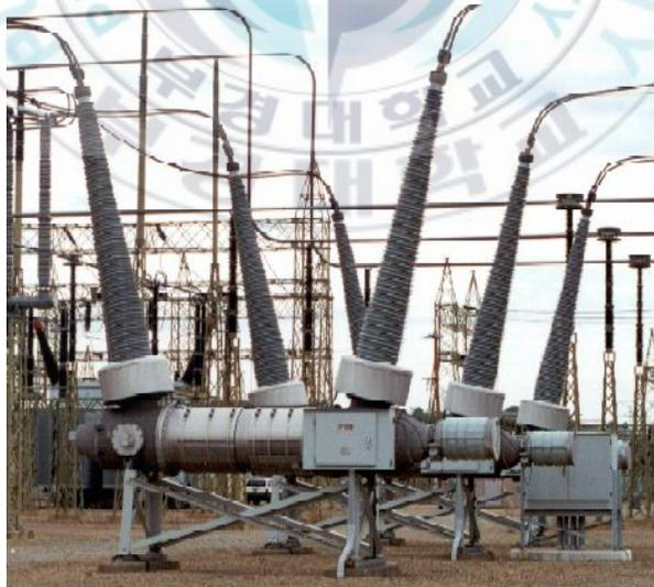
Fig. 2.1 Oil pressure type circuit breaker.
