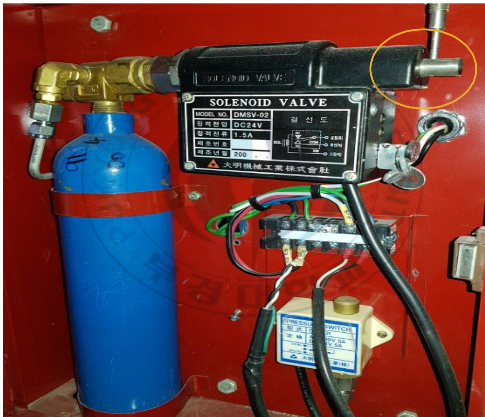
Photo 1. Locking pin installed on solenoid valve.
