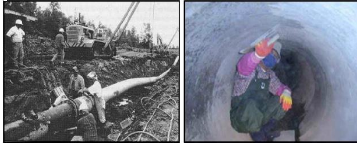
Fig. 1.2 Manual inspection and maintenance of pipe
