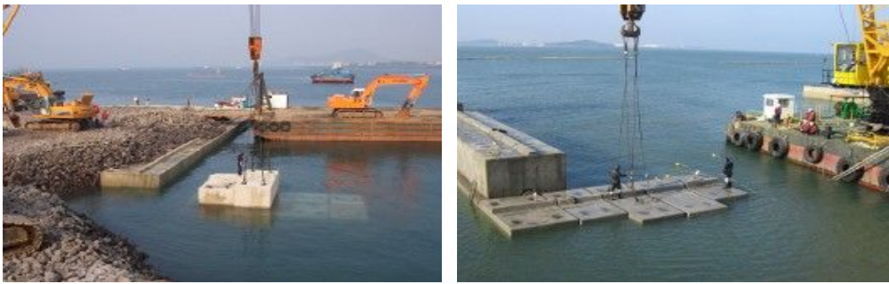
Fig.4 Block installation of above water
