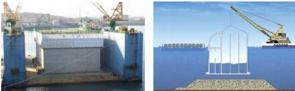
Fig.1 Caisson fabrication and installation
