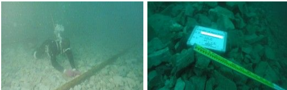
Fig.3 Leveling of foundation and armor stone
