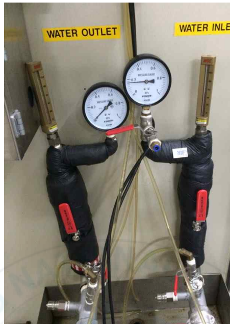
Figure 3.5 A part of the test facility for the support and recovery of water to the test models of the fin-tube radiator.
