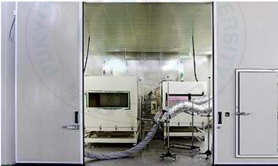
Figure 3.1 30 refrigeration ton humidity chamber used for estimation of the heat transfer performance of the test models of the fin-tube radiator.
