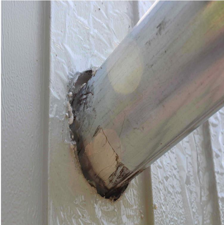
Photo 9 Styrofoam area are dissolved by the heat of the chimney.
