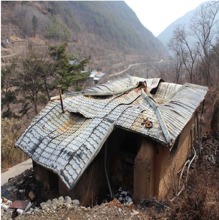
Photo 6 Roof figure appears curvature phenomenon by heat.
