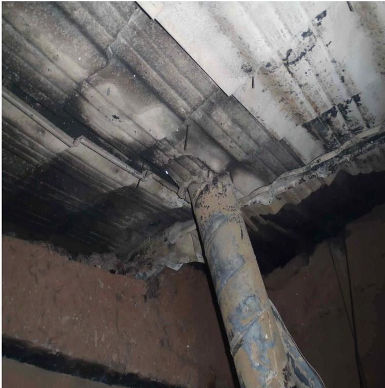
Photo 5 Combustion trace from folding part of stovepipe and roof.
