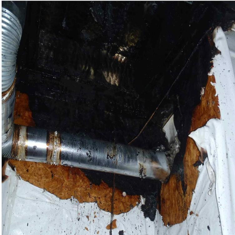
Photo 1 The firing pattern which combusted from top of the stovepipe.
