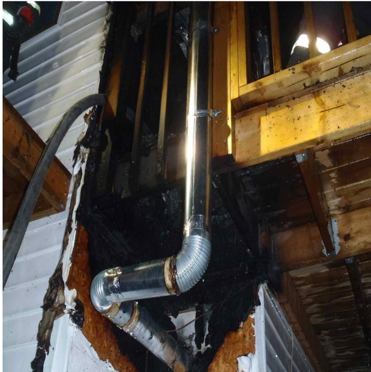
Photo 2 The firing pattern combusted upper side along the external wall.
