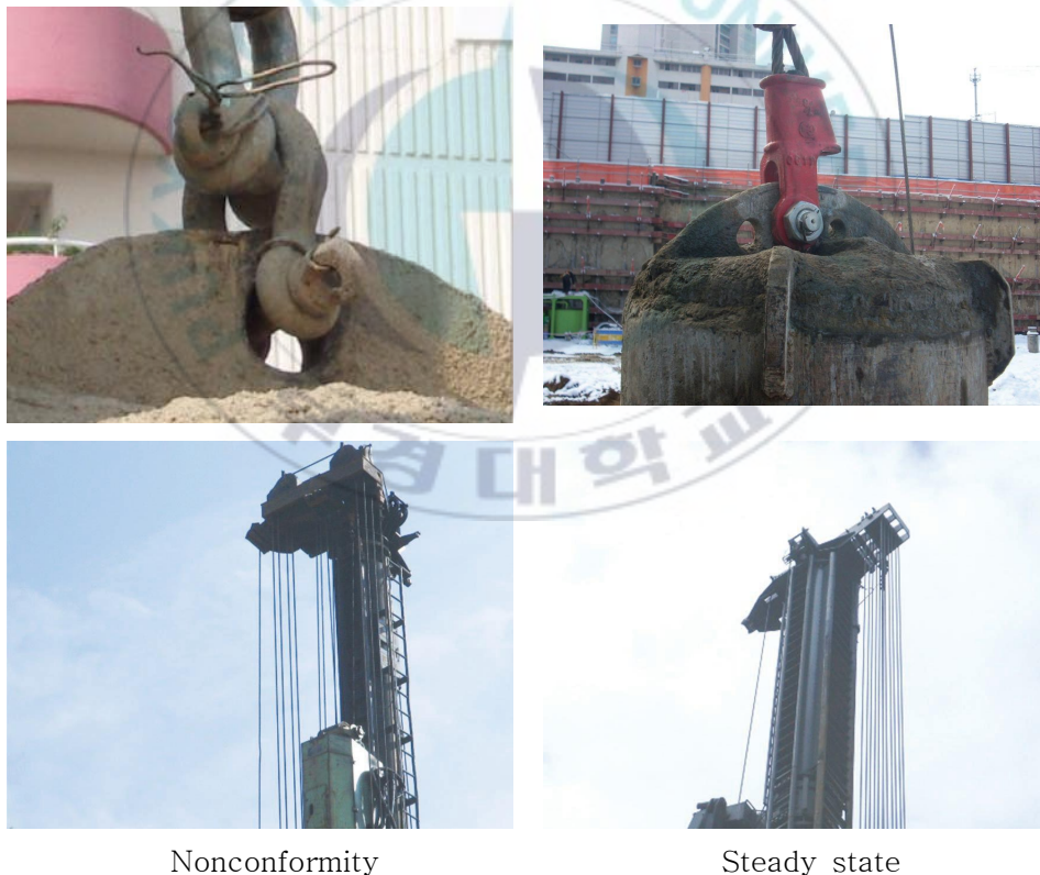
Fig. 2.9 Problems of hammers and winding and preventing devices[36]
