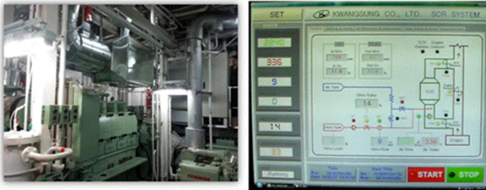
Fig. 11. Picture of SCR system in Kaya ship
