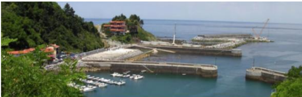
(c) Mutriku OWC breakwater
