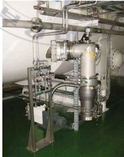
Fig. 2.8 Vacuum pumping system
