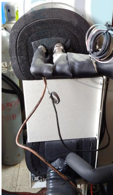
Figure 13 Intermediate heat exchanger
