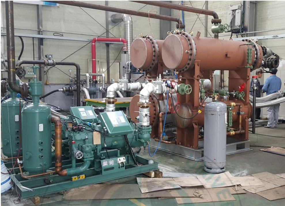
Figure 7 Experimental apparatus of seawater cooling system [12]
