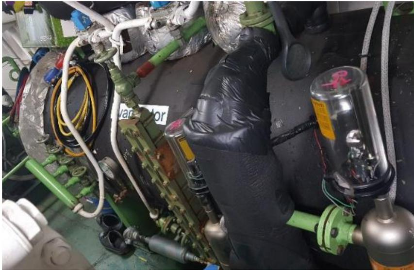
Figure 16 Condenser installed in the fishing vessel [12]
