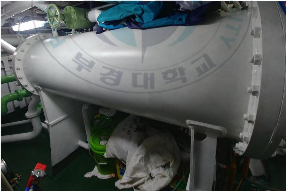
Figure 15 Condenser installed in the fishing vessel [12]
