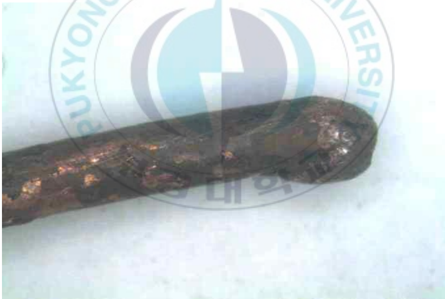
Photo 8. Appearance of bead by short-circuit on the solid wire separated wires of the wall-mounted fan found at the restaurant.
