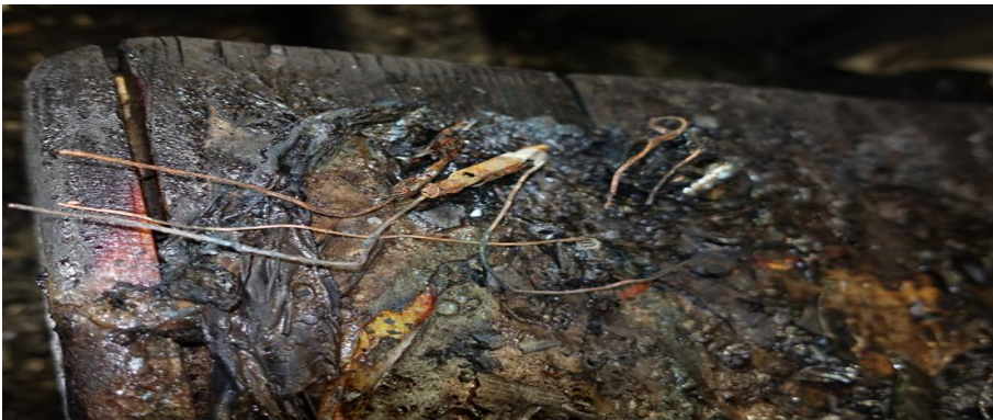
Photo 1. Identification of the spark on the damaged connection wiring of hand drill charger.
