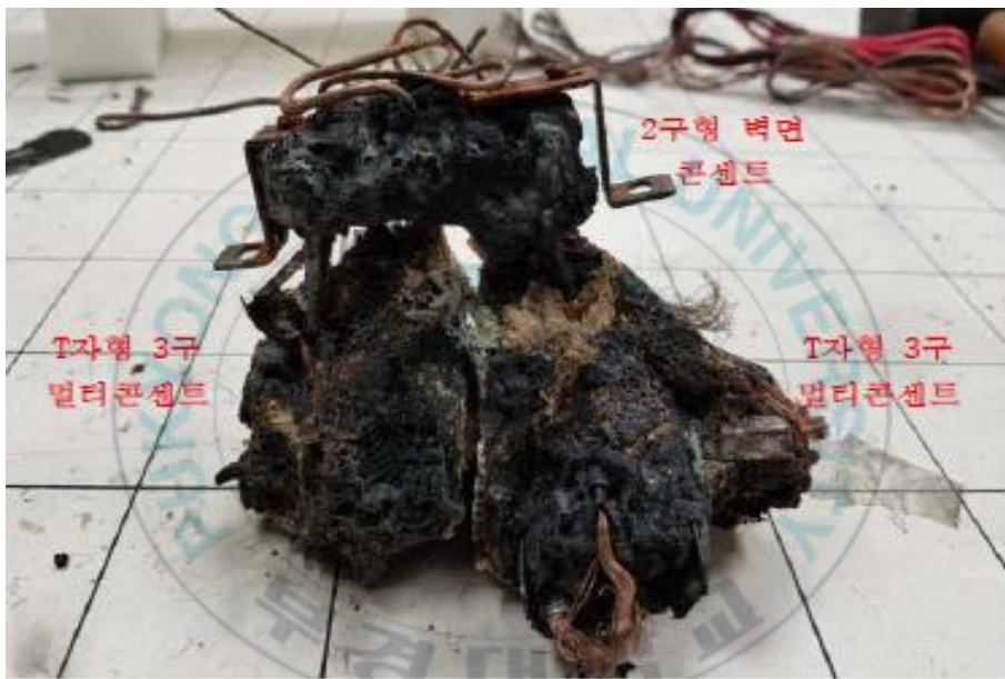
Photo 7. A 2-prong wall outlet and a T-shaped 3-prong multi-outlet are combined lost in state.
