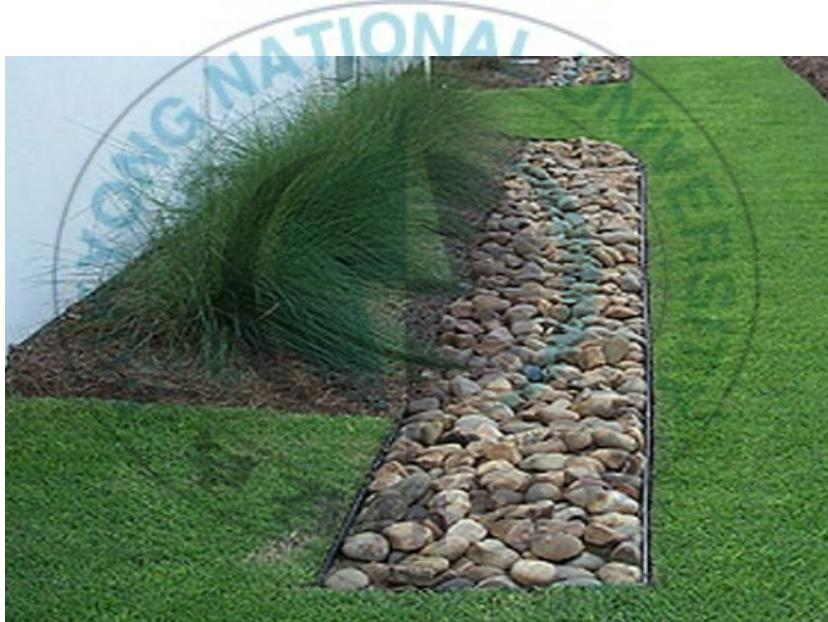
Fig. 2.15 Infiltration Trench.
