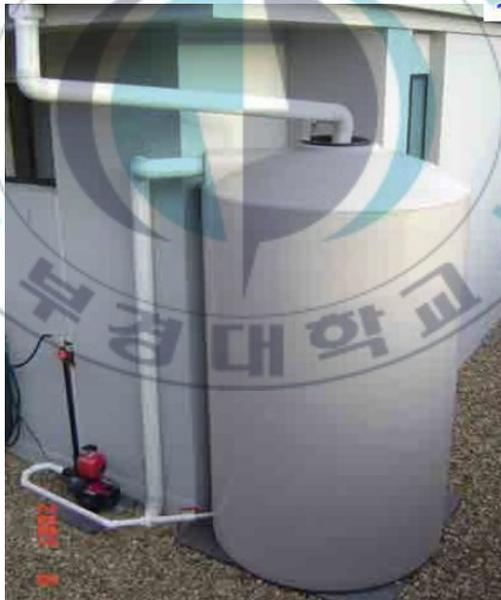
Fig. 2.17 Rain Barrel.
