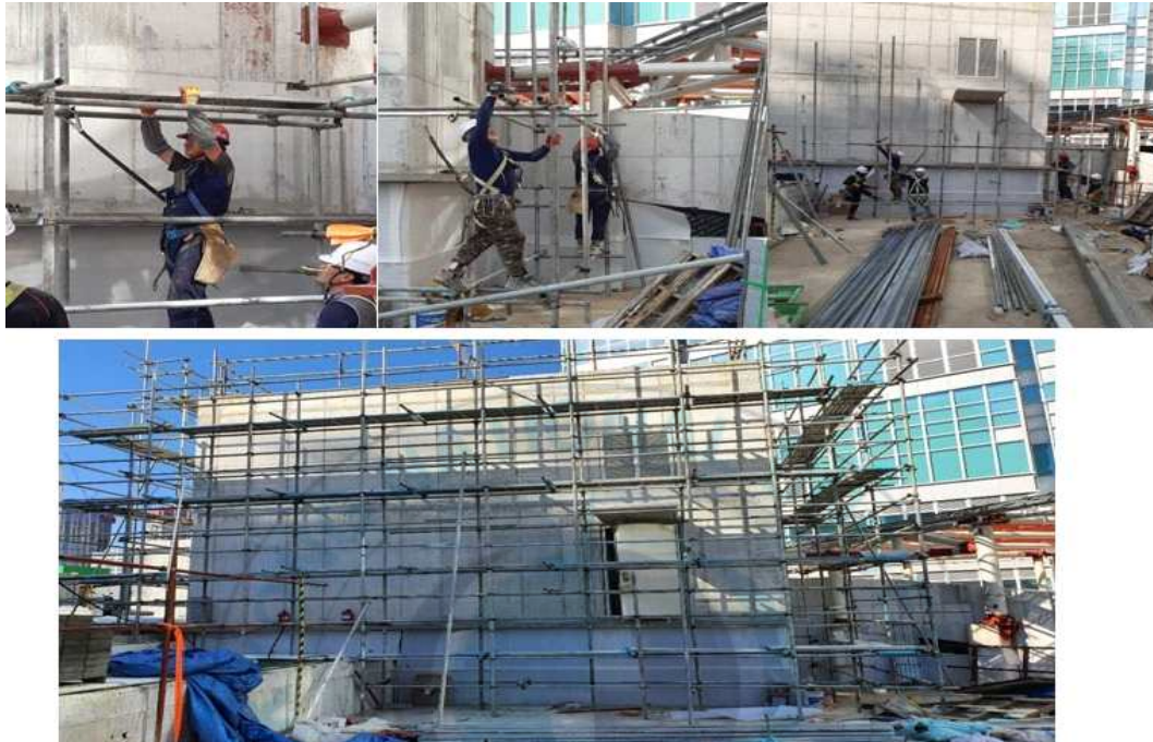
FIG. 2.4 Scaffolding installation work and completion status [2]
