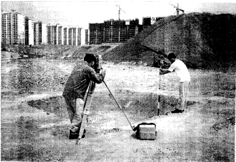
Fig. 3.9 Measurement by Total Station
