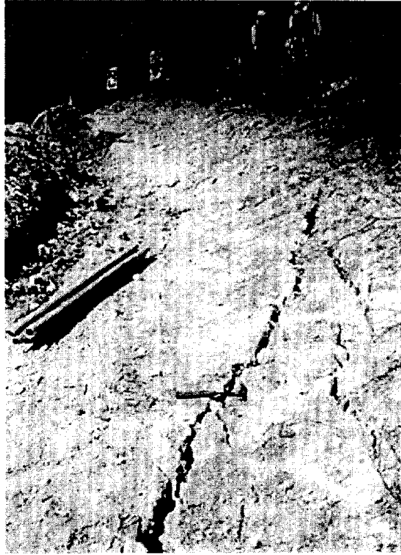
Fig. 27. More extended tension cracks in upper drainage.
