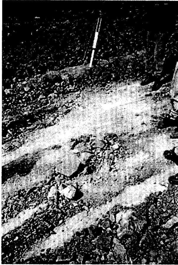
Fig. 29. Exposed slide plane(about 12° dip).
