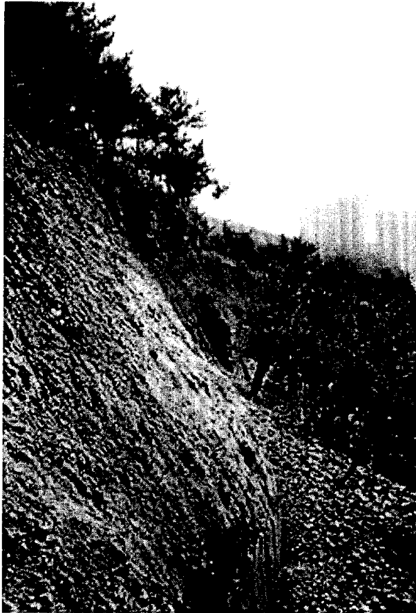
Fig. 22. Vertical failure plane occurred the first landslide.
