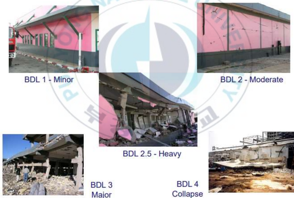
Fig. 3. Building Damage Level (BDL) Categories (Examples) 18)
