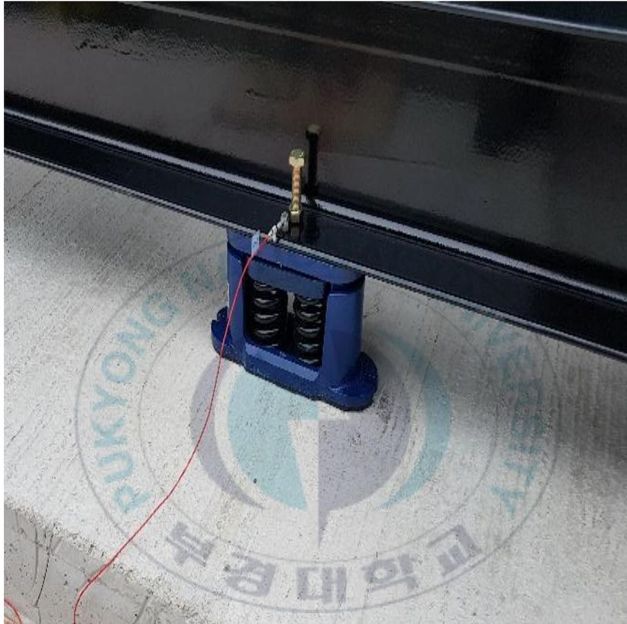
**Figure 3** Passive-type mount module of emergency electric generator including basement mass-block<sup>(3)</sup>
