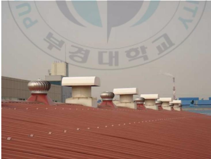
Fig. 3.3 Natural Ventilator with Power Fan
