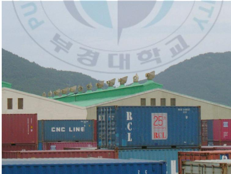
Fig. 3.7 Roof Monitor with Natural Ventilator
