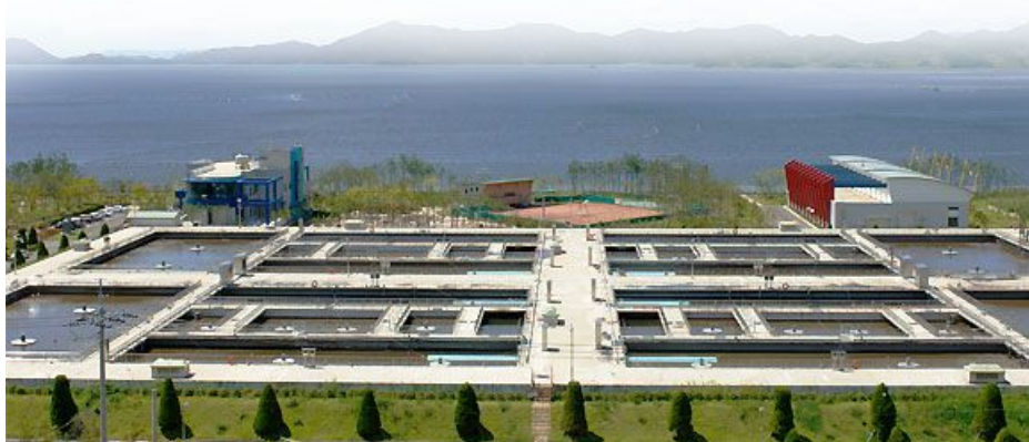
Fig. 23. Overview of Yeosu sewage treatment plant in Gamak Bay (Yeosu City, 2007)
