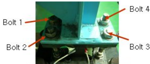
Fig. 6.9 Bolts Connecting Girder to Support System
